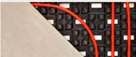
Pouring filling compound.
