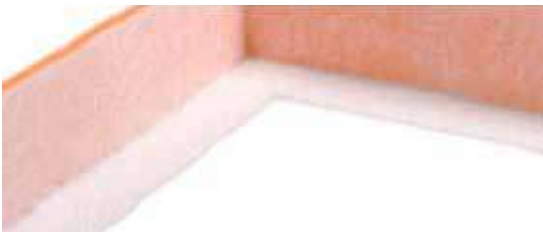
Fixing insulation strip to walls.
